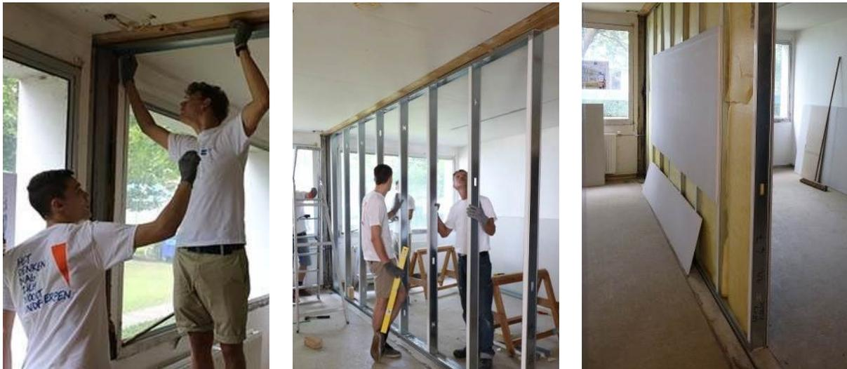
Figure 22: Construction of the Wall-LinQ system, based on metal profiles, during the summer school
