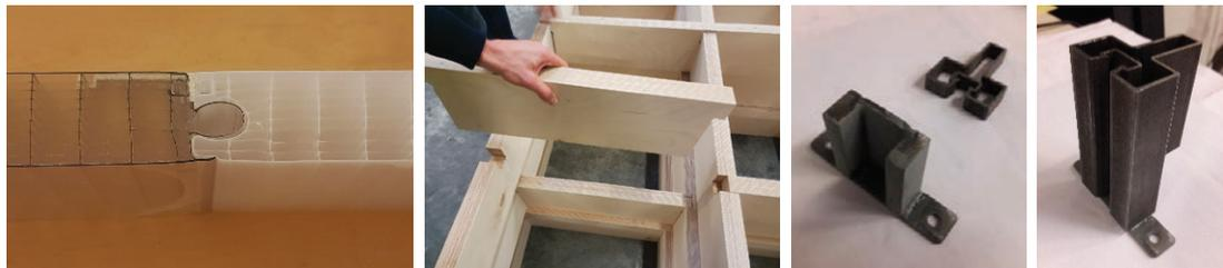
Figure 55 Examples of interlock connections.
