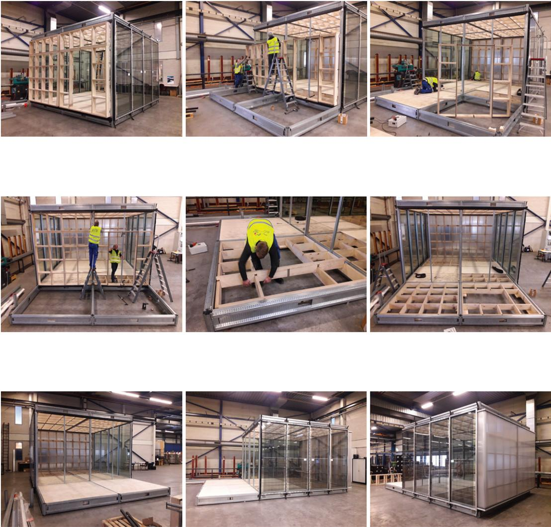
Figure 70 Transformation and extension of GTB Lab module
