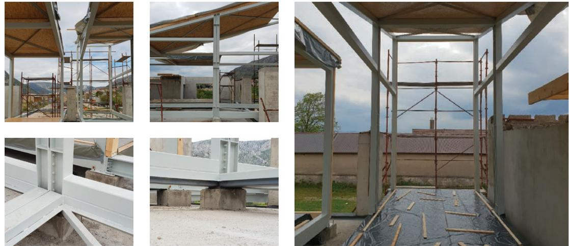
Figure 79 Mounting the reversible floor and roof elements on the steel frame
