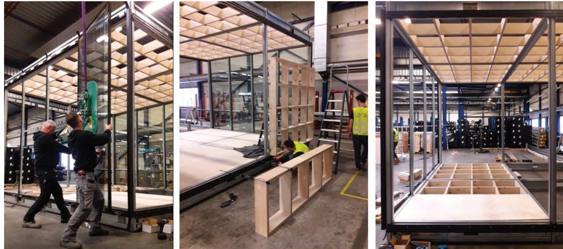
**Figure 53** illustrates gravity principle of assembly. All parts can be assembled in parallel and create connection only with the main frame. (GTB Lab module)
