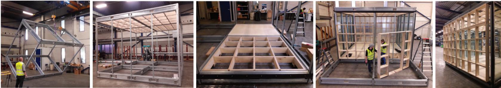
**Figure 49** Assembly of the steel frame which functions as a base for other clusters as façade, roof floor. All are independently produced and assembled independently from each other (GTB Lab)
