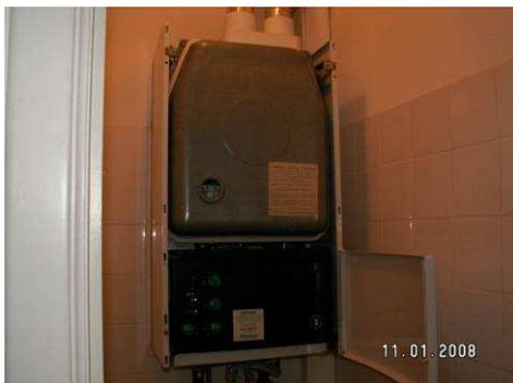
Figure 7.21: chaudière murale au gaz (type C)
