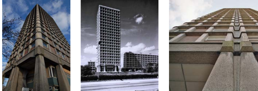
Figure 5.14: Tower at Boom before renovation
