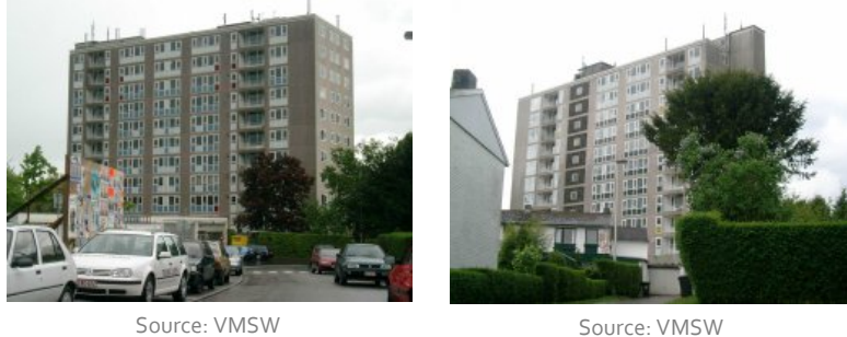
Figure 5.12: Sterrenveld and Zonneveld before renovation (Ban Eik - Wezenbeek-Oppem)
