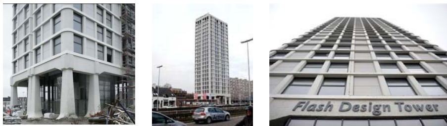
Figure 5.16: Tower at Boom after renovation
