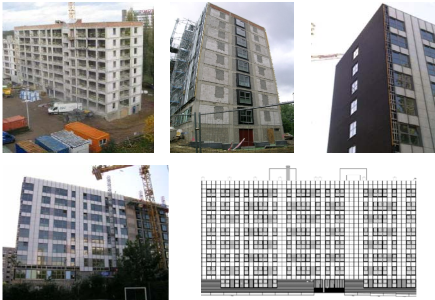
Figure 9.4: Building block IX during and after renovation
