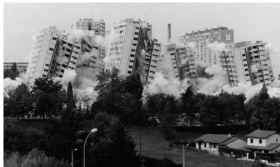
Figure 2.4: Demolition of les Minguettes near Lyon (France)
