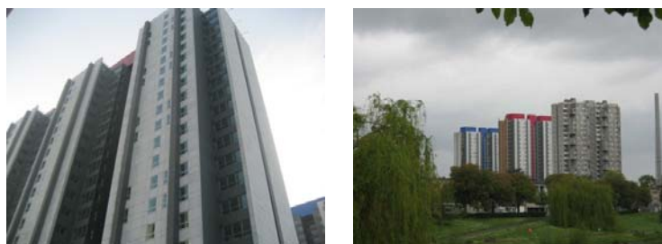
Figure 5.11: Silvertop tower after renovation
