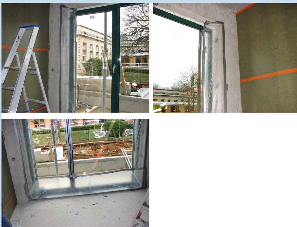
Test in situ (Source : DEL Expertises sprl)
