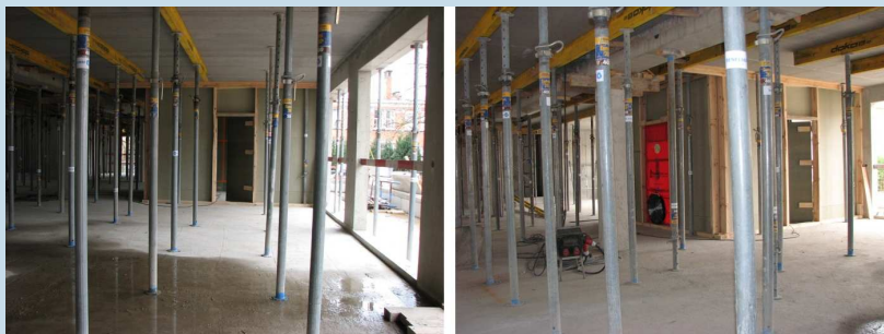
Test in situ (Source : DEL Expertises sprl)
