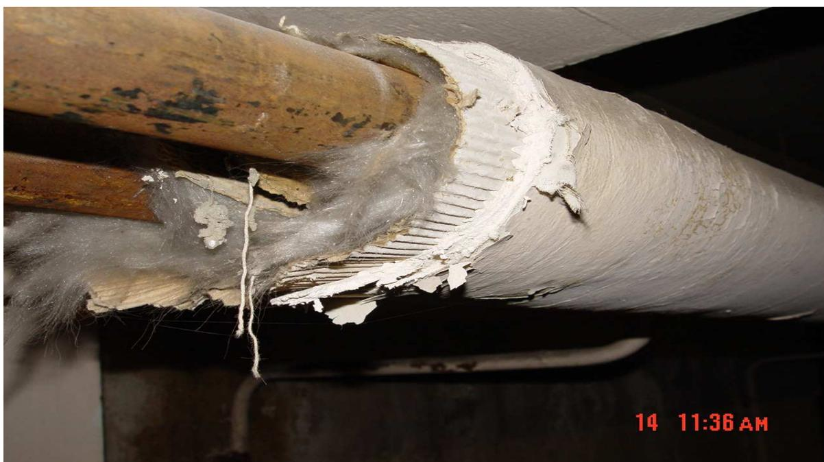
**Figure 4.3.4: Isolation thermique**
