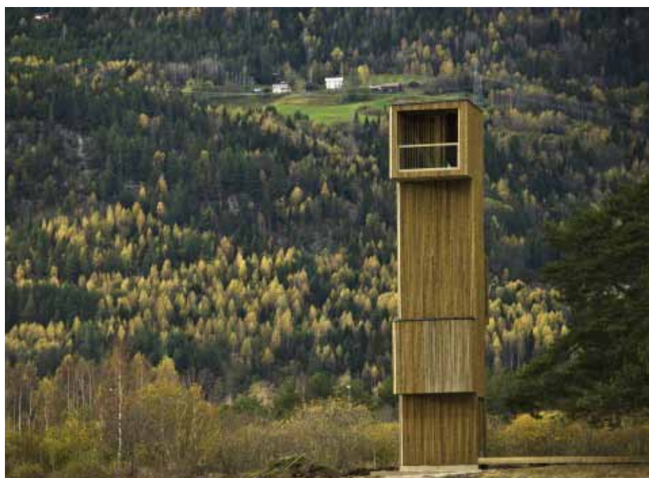
Rintala Eggertsson Architects Selyord Lookout Point
