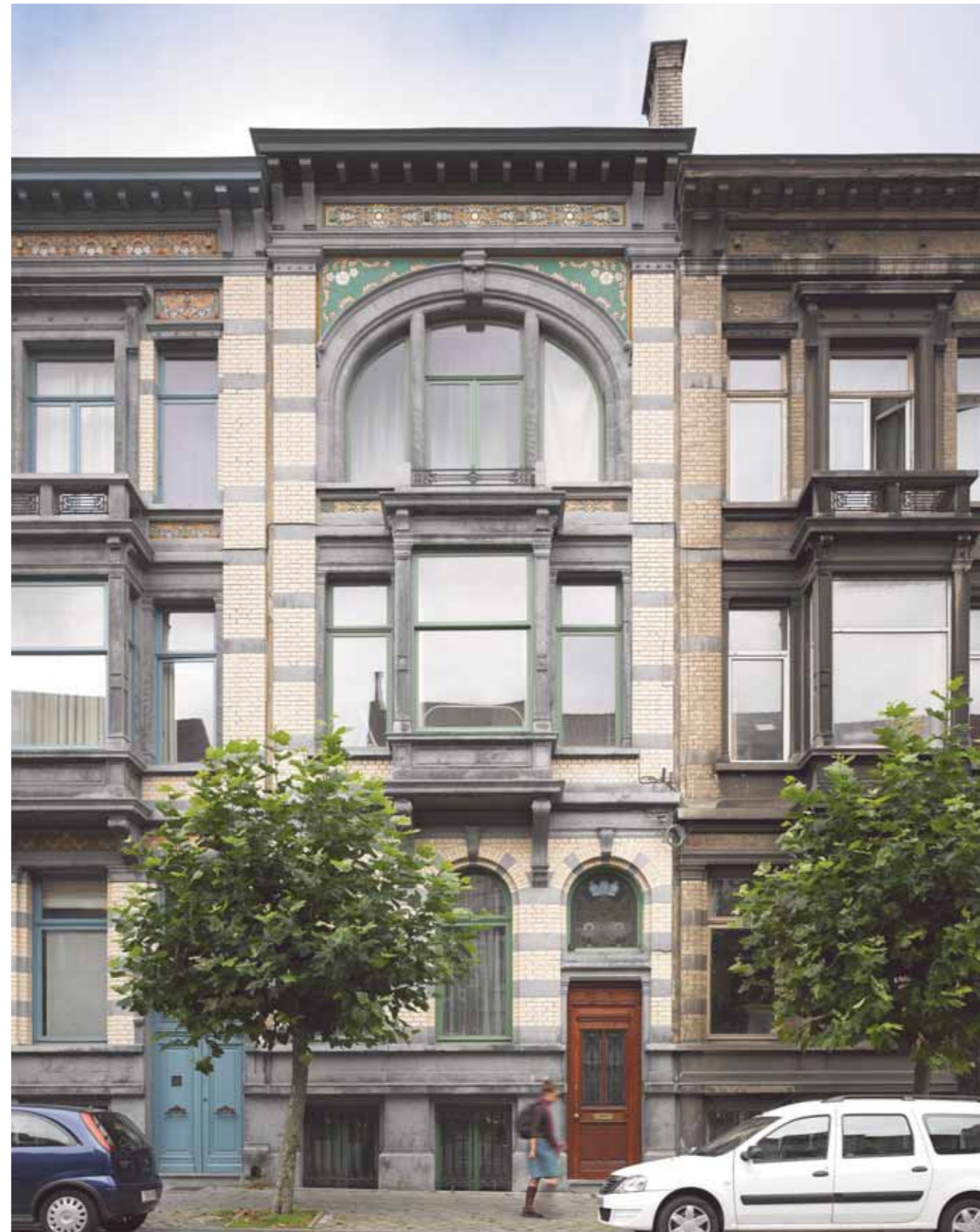
Renovation of a building on Rue Royale Sainte-Marie [099]: the project has renovated the 3 upper levels of a typical Brussels house to produce 3 dwelling units. Using mostly natural materials, expert craftsmanship was needed to incorporate the insulation and ventilation into the existing eclectic architecture. The existing window frames have been maintained and repaired (P. Abel, architect).
