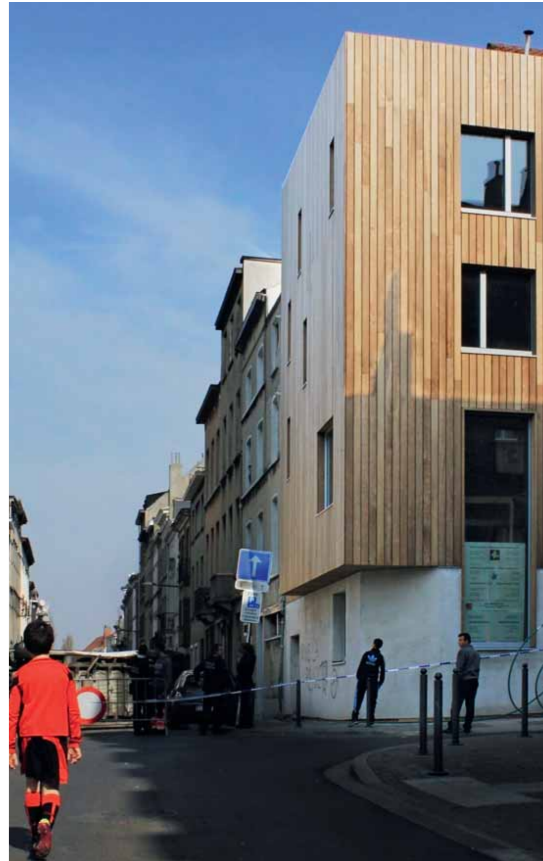
Public housing passive on Rue de la Poste [087]: the reconstruction of the housing unit on Rue de la Poste has been done with a wood frame in order to reuse the existing building foundation (CMDN architecture).
