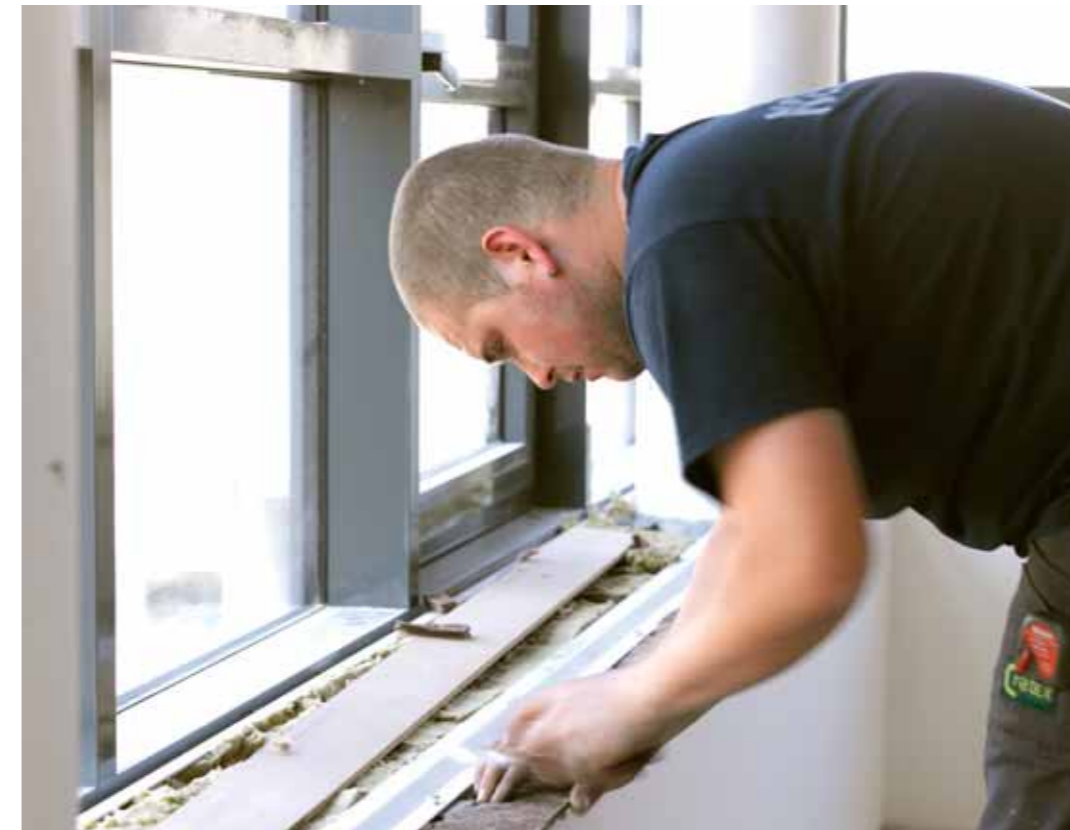
Renovation and heightening of a building on Rue de la Loi [068]: the architects used a prefabrication method which unfortunately did not distinguish walls needing to be airtight from the other walls. Corrections had to be made on site, which proved more difficult than planned, even if the n50 value is nearly reached today (Synergy international).
