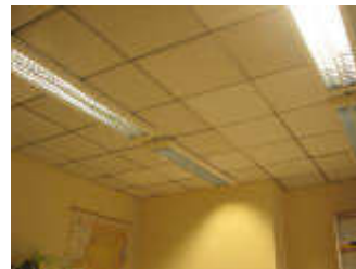
Relighting kantoor > 1300 lux (norm: 300-500 lux)
