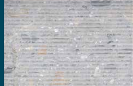
Diamond grinding beton
