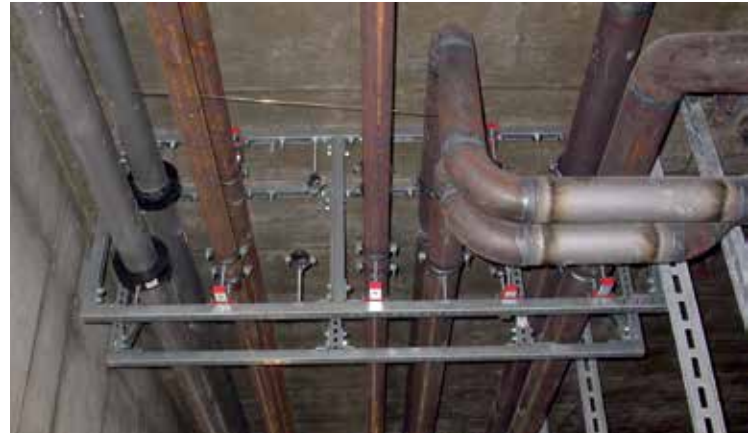
Figure 24: Support Quick Assembly & Disassembly - wall mounting systems allow quick installation & removal of products fixed to walls. Photo Würth, Künzelsau.
