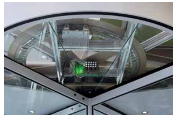
Figure 31: Kinetic Energy: An Unusual Highlight—energy-generating revolving door at Natuurcafé La Port, The Netherlands (left) and detail of kinetic mechanism (right). Photos Boon Edam.
