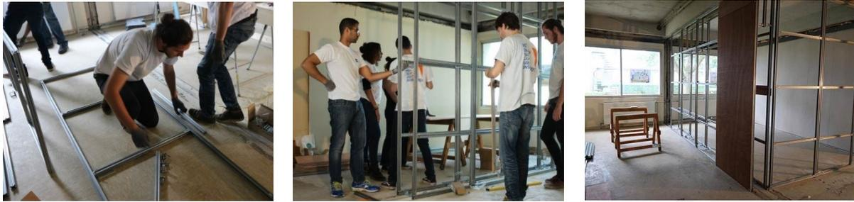
Figure 19: Construction of a partition wall with integrated desk and bookshelves created with the Geberit GIS system during the Summer School (finished with plywood panels)
