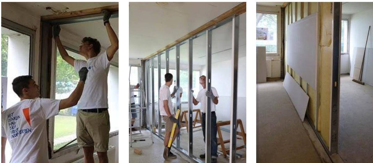
Figure 22: Construction of the Wall-LinQ system, based on metal profiles, during the summer school
