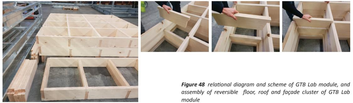
**Figure 48** relational diagram and scheme of GTB Lab module, and assembly of reversible floor, roof and façade cluster of GTB Lab module
