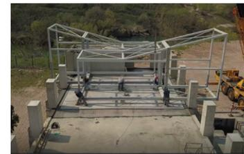
**Figure 78** *Placing reversible steel frame on the existing structure*
