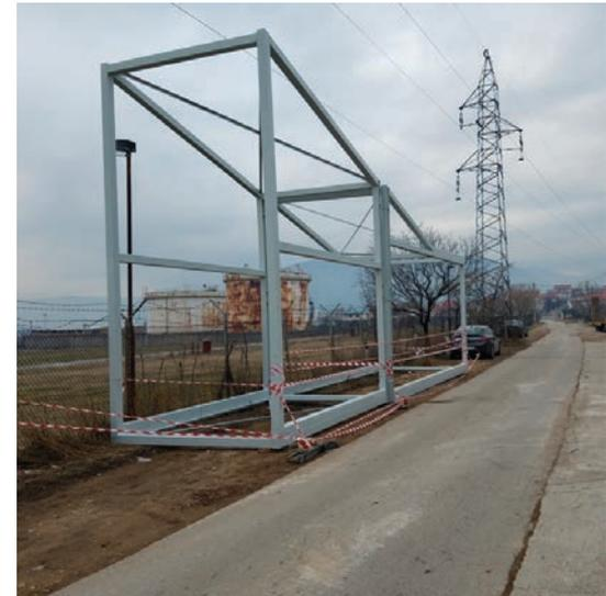
Figure 77 Prototype of the steel frame
