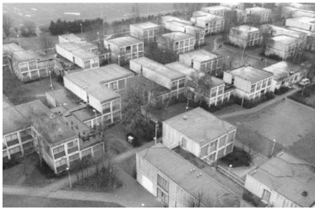
Figure 43: VARIEL System at VUB
