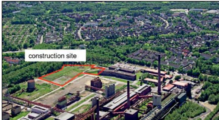
Figure 34: Construction site on “Zeche Zollverein” Essen, Germany.
