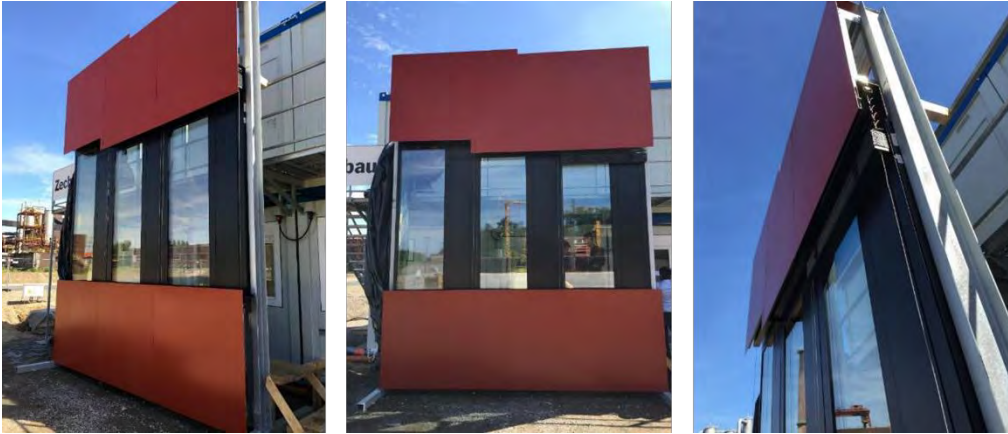
Figure 84: New Office Building – Facade module
