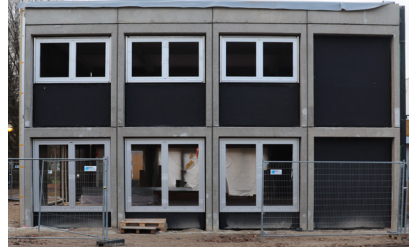
INSULATION WATERPROOF PANELS INFILL
