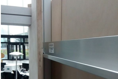
Detail of horizontal, vertical and orthogonal profiles and the birch panel
