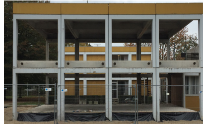
STRIPPED CONCRETE STRUCTURE
