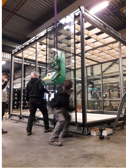
Assembling reversible triple glass panels with PV strips produced by Pilkington in Enschede NL.
