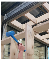
Assembling reversible triple glass panels with PV strips produced by Pilkington in Enschede NL.
