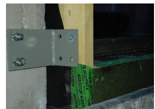
CIRCULAR RETROFIT LAB
