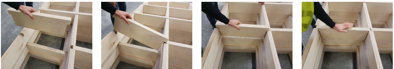
Three dimensions for Steel intermediary elements had been specified. In the first place, the industry produced only one dimension. In order to avoid waste by producing all new connectors a decision was taken to add an additional wooden intermediary under the floor cassettes and use already manufactured elements as much as possible to connect the steel frame with the roof, floor and facades.
