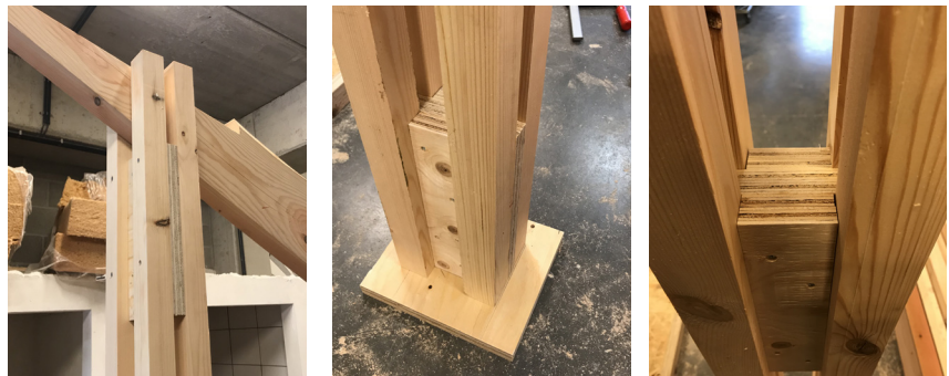
Figure 27: The columns were constructed during the EFP workshop in the winter 2018
