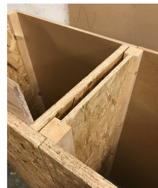
Figure 34: The insulated cassettes for the facade system were realised in the EFP workshop during the winter 2018
