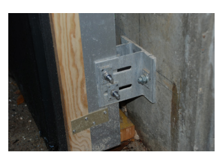
CIRCULAR RETROFIT LAB
