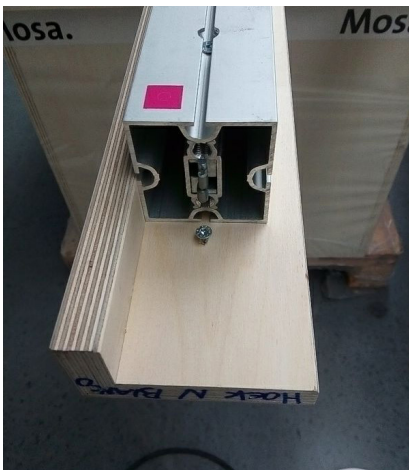
Detail of corner of horizontal Octanorm profile and birch panels with custom screw-connector
