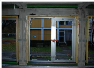
CIRCULAR RETROFIT LAB
