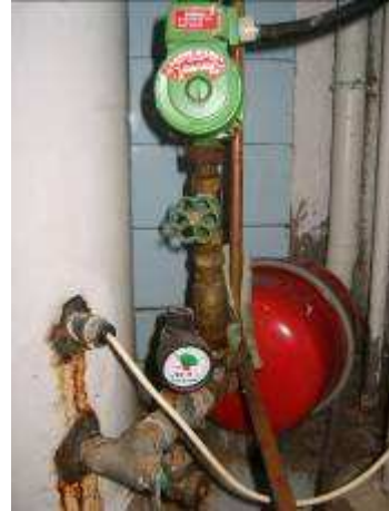
Figure 5. corrosion du ballon
