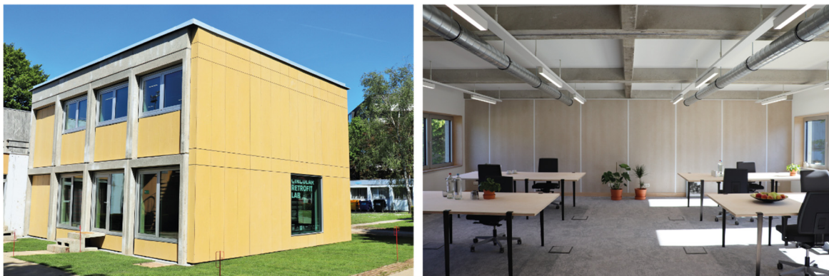
Figure 2. The Circular Retrofit Lab is a set of refurbished student housing modules, currently housing a dissemination space and offices.
